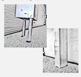
2. Slide base tube pins into holes in concrete.
