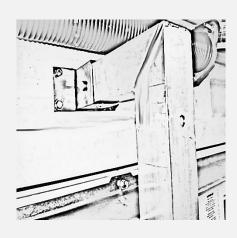
3. Extend telescoping end above door, sliding into bracket. Push bolt through post and pin in place.
