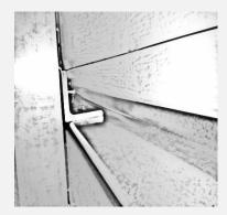
4. Align bracket (s) on door struts (Ubars) and attach using bolt and pin.
